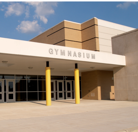
Public non-residential building (school)
