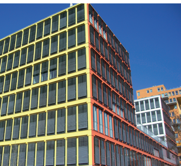
Non-residential building (office)
