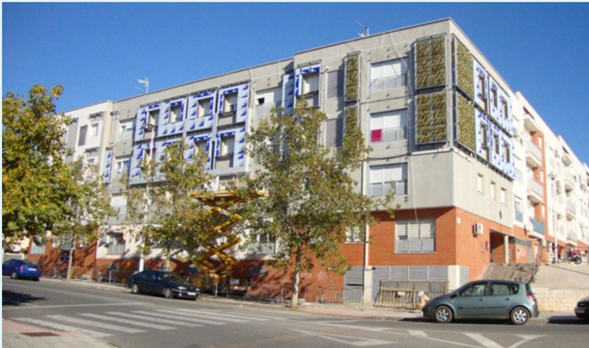
Figure 20 – Smart facades in Merida in Spain (Source: MEEFS Façade concept [35], 2015)
